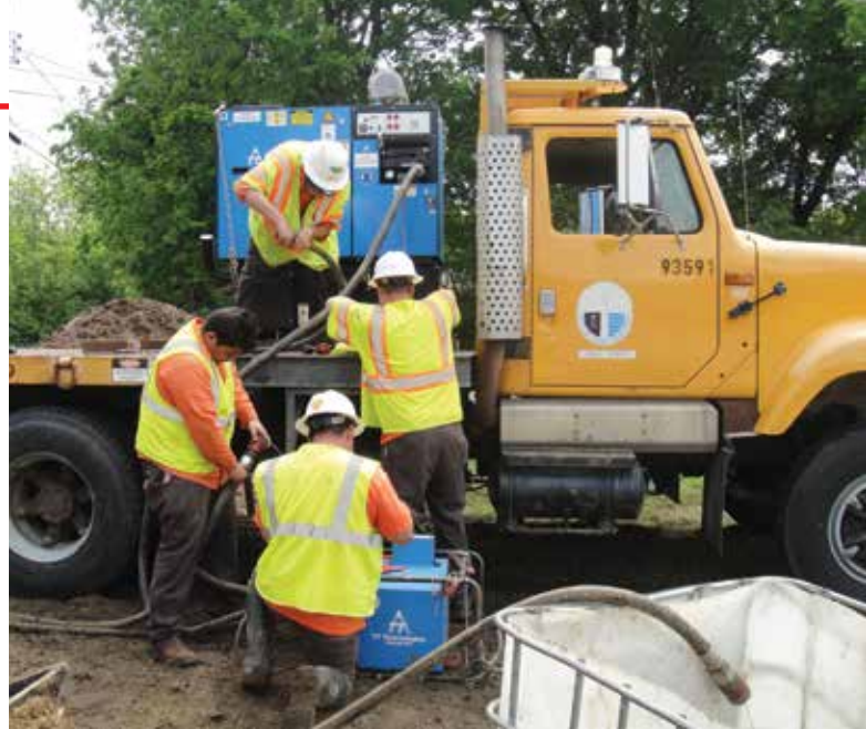
City crews enjoy working with all of Tulsa's trenchless technology equipment
