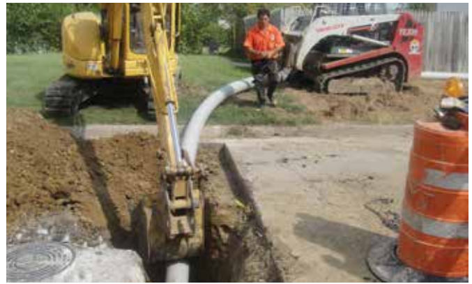
Majority of Tulsa's slip-line work involves inserting 7.125-inch DR 19 HDPE pipe
